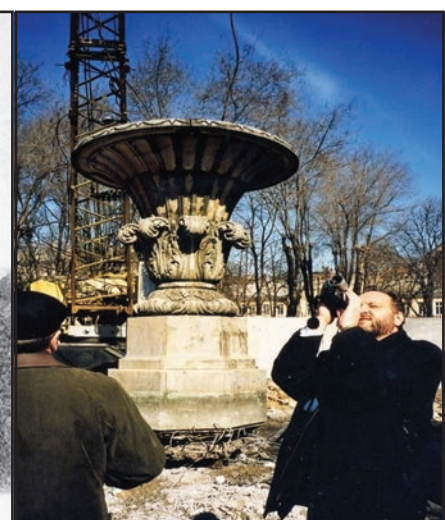
Fig. 2. Dismantling of the marble bowl of the Filatov's fountain. The photo by Mechsheriakov V.N., March, 30th, 2001 [11].
