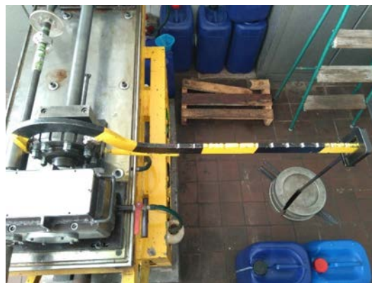
Fig. 3. Three-phase electric motor of Niemann M01
