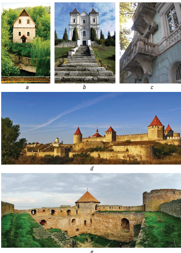
Fig. 1. The buildings and structures built of limestone-shell rock: a – Water Mill (Stroenets, Moldova); b – Church of St. Cajetan (Rashkov, Moldova); c – House of Marazli (4, Pushkynska str., Odessa, Ukraine); d – Bendery Fortress (Moldova); e – Akkerman Fortress (Bilhorod-Dnistrovsk, Ukraine)
