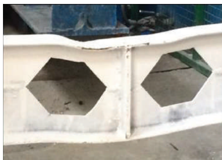
Fig. 7. Failure mode of specimen CBN-0
