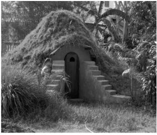
Fig. 5. Example of earth-bag construction
