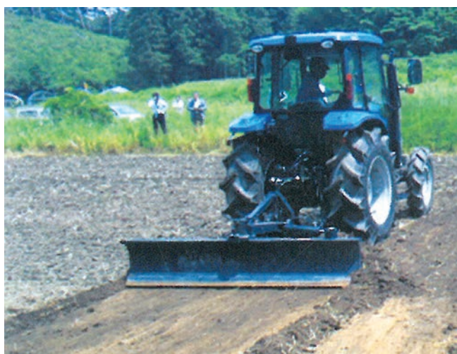
Fig. 2. Upper contaminated ground layer removal (Japan)
