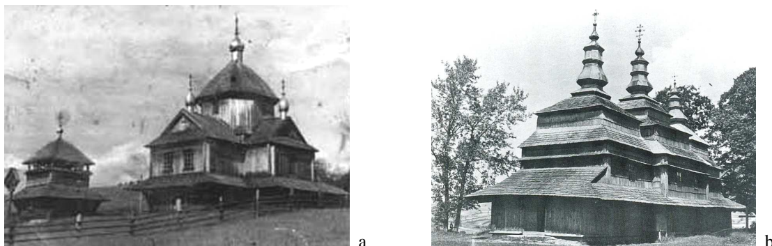
Fig. 3. Non-existent woden churches destroyed after the deportation of Ukrainians (in 1947) in Tisna commune: a) The church of St. Mykolay Chudotvorets from 1830 with a bell tower with “one dome” structure in Dovzhytsya, b) The church of the St. Martyr Dmytryj from 1875 with three-sector form and “three dome” structure in Smerek
