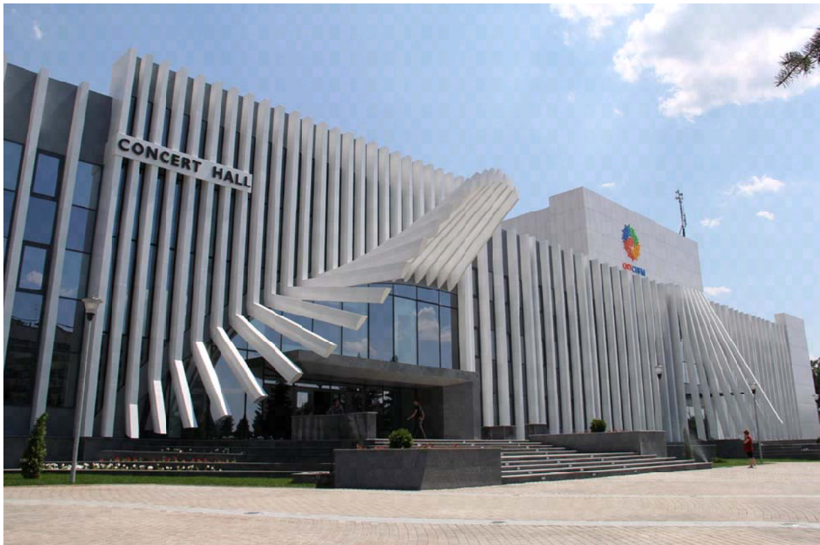
Figure 1. General view of the building after refurbishment (facades 1–19).
