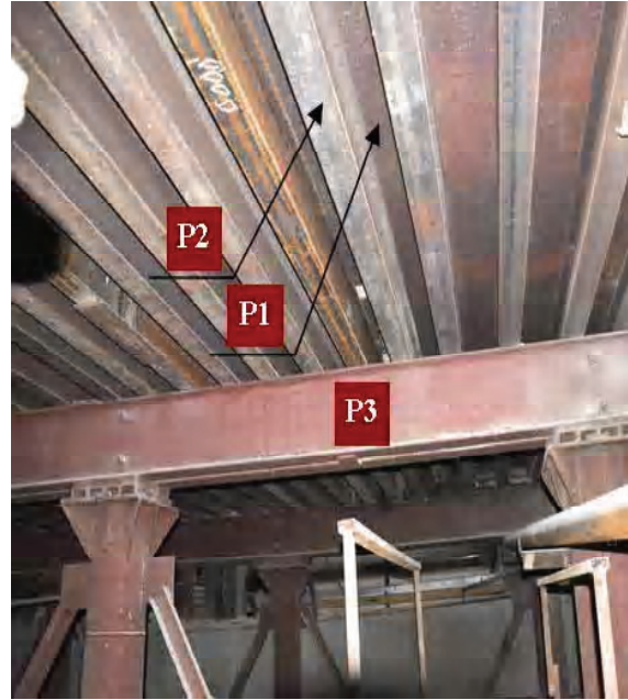
Figure 4. The points of the bottom temperature control.
