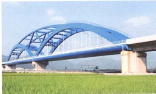
(c) Yandangshan Bridge
