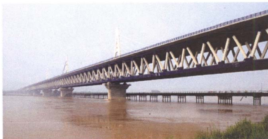
(c) Zhengzhou Bridge
