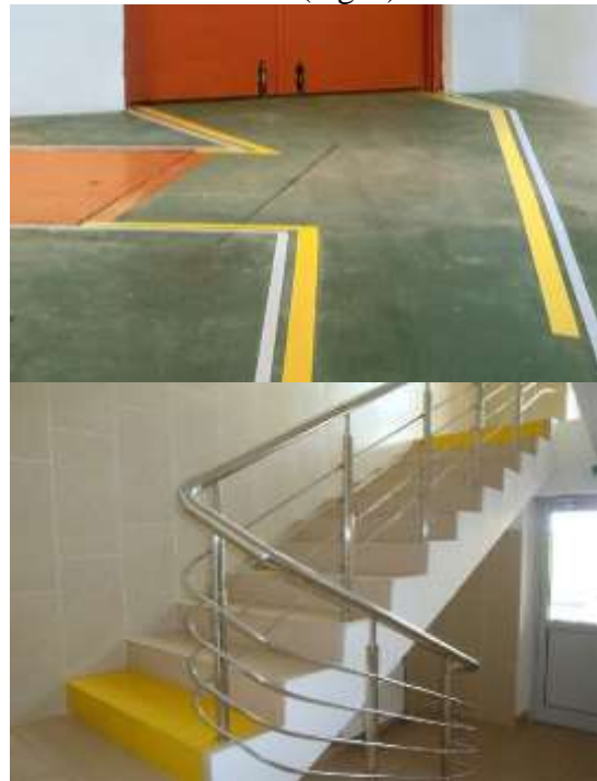
Fig. 3. Examples of color scheme of a marking of horizontal and vertical communications
