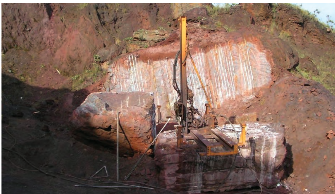
Fig. 2. Mining jaspilites with the string drilling machine application, Brazil [7]
