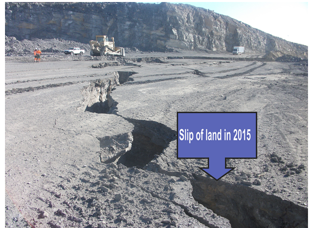
Fig. 3. Quarry of Chouf Amar after sliding [6]
