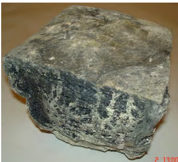
Fig. 2. A sample of concrete with applied polymer compound coat based on the secondary materials after testing under the corrosive environment conditions in camera No. 2 of the sewer in Kharkiv
