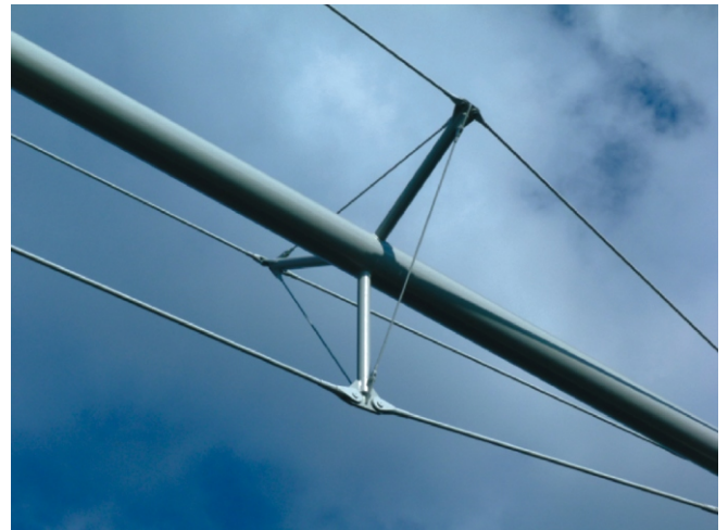
Fig. 7. Cross-frame beam – spatial beam string structure
