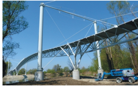
Fig. 13. View on steel structure
