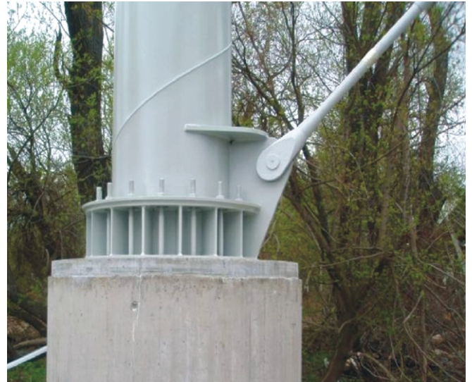
Fig. 5. Anchoring of the pylon – proposal and realization
