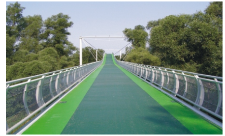
Fig. 14. View on finished bridge
