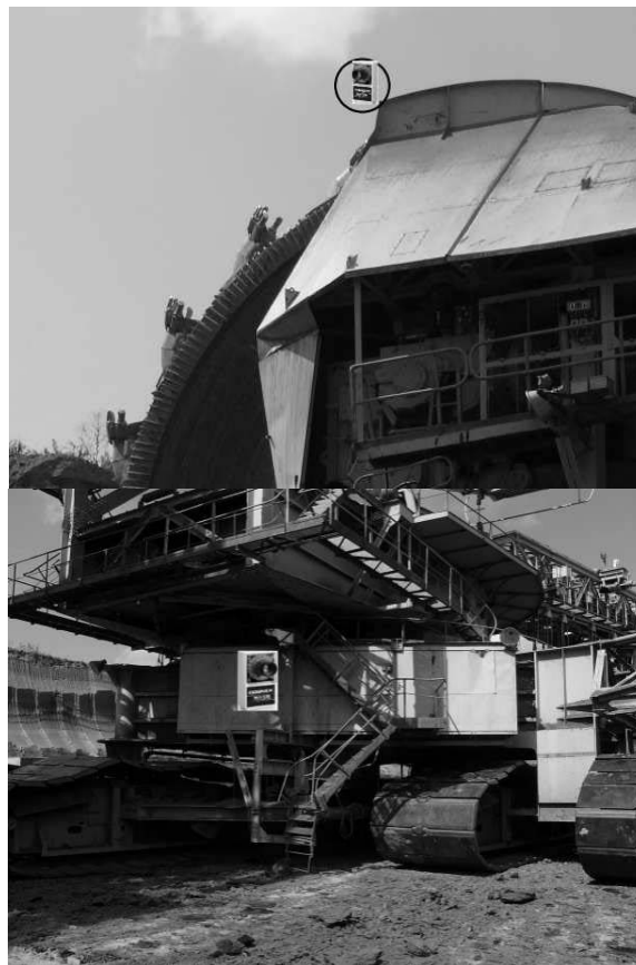
Fig. 6. DVT Vision sensor positions on the bucket wheel excavator
