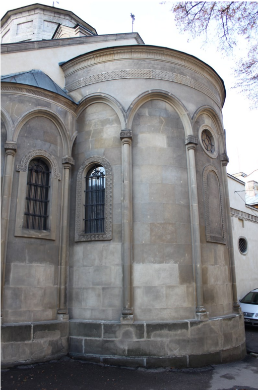
Photo 2. Basement of the ancient buildings of Lviv City made with trim sandstone (a) and limestone (b) blocks
