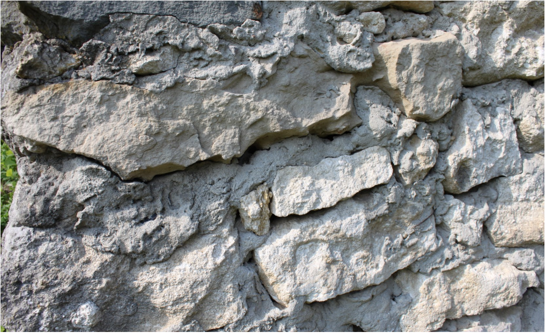
Photo 1. Fragment of the basement of rocky defensive tower near Piatnychany village
