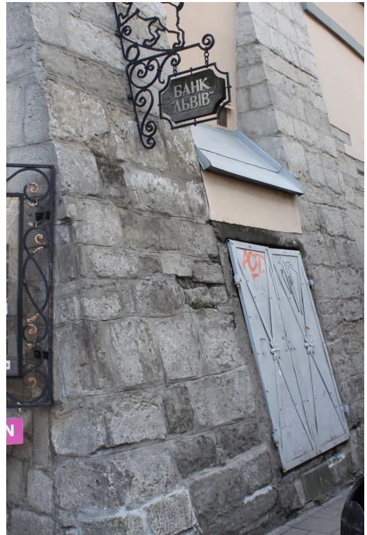
Photo 2. Basement of the ancient buildings of Lviv City made with trim sandstone (a) and limestone (b) blocks
