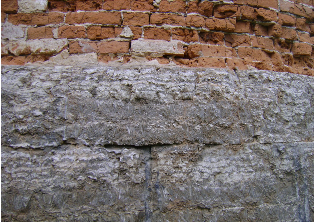
Photo 4. Basement of the Assumption Cathedral Church in Krylos Village made with trim alabaster blocks (a) and fragment of the trim gypsum basement (b) of the Earl's Ray Palace in Pryozerne Village
