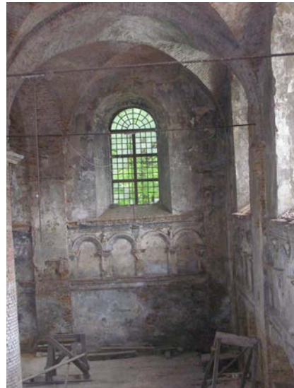
Fig. 20. Fragment of interior of the synagogue that includes an extreme window, of which axis does not coincide with the axis of the vault: photo taken in 2008.
