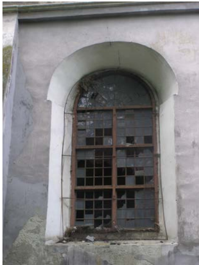
Fig. 19. Traces of lowering of a window on the northern facade: photo taken in 2008.
