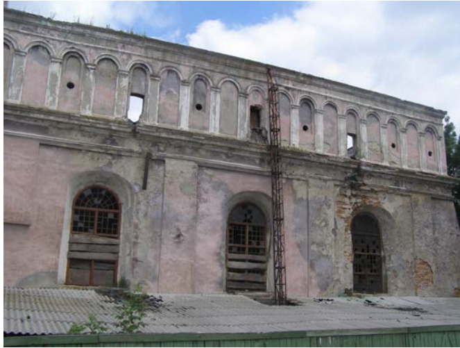
Fig. 18. Synagogue in Zhovkva. Southern facade. Openings in the windows reveal signs of lowering: photo taken in 2008.
