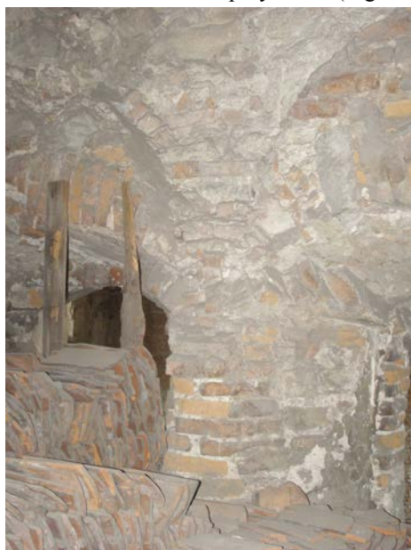
Fig. 9. Traces of rebuilding of wall of the western synagogue's body: photo taken in 2008.
