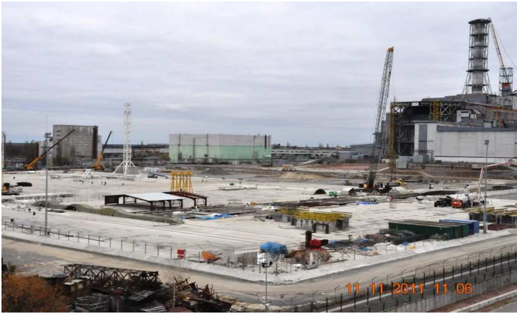
Platform for Arch assembly, November 2011
