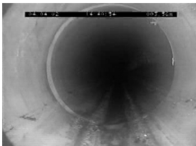
Fig. 14. One sided longitudinal displacement in the 5th class
