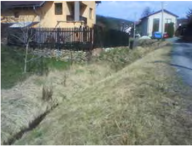
Fig. 7. Creek in Vydrník village – initial state
