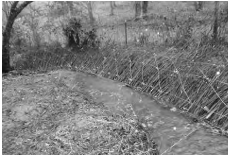
Fig. 1. Installed brush mattress
