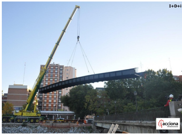
Fig. 1. (a) Installation of the FRP girder; (b) View of the Almuñecar footbridge (Courtesy of Acciona Infr.)
