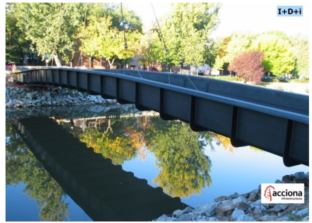
Fig. 1. (a) Installation of the FRP girder; (b) View of the Almuñecar footbridge (Courtesy of Acciona Infr.)
