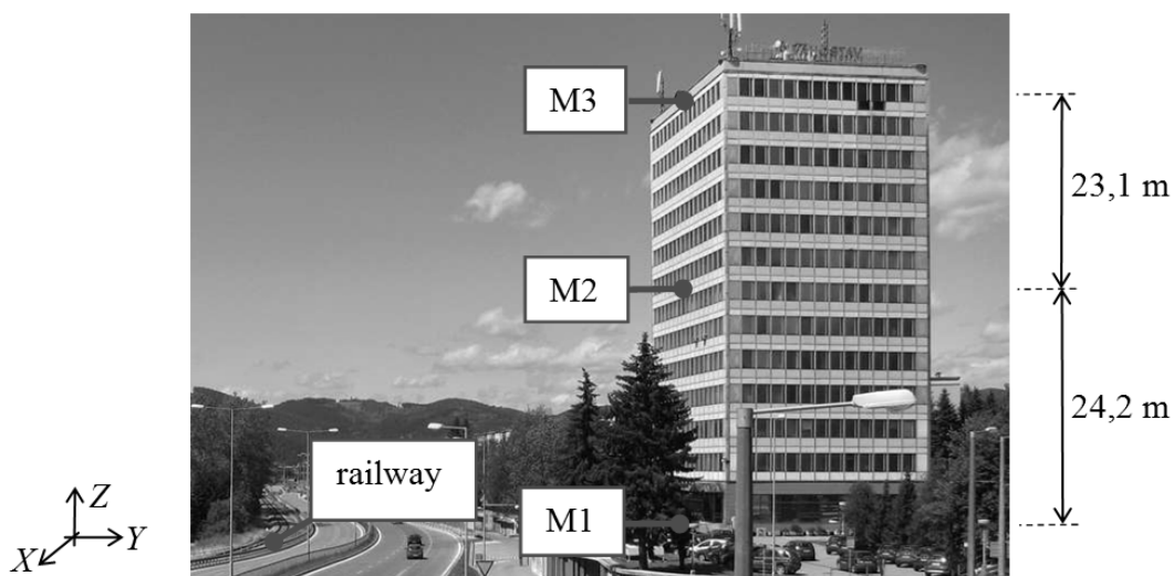
Fig. 1. Situation of reinforced concrete building and railway line, Distribution of measuring points: M1 – basement; M2 – 7. floor; M3 – roof
