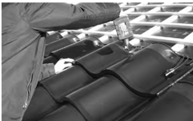
Fig. 2. Roof tiles with integrated solar photovoltaic cells [10]
