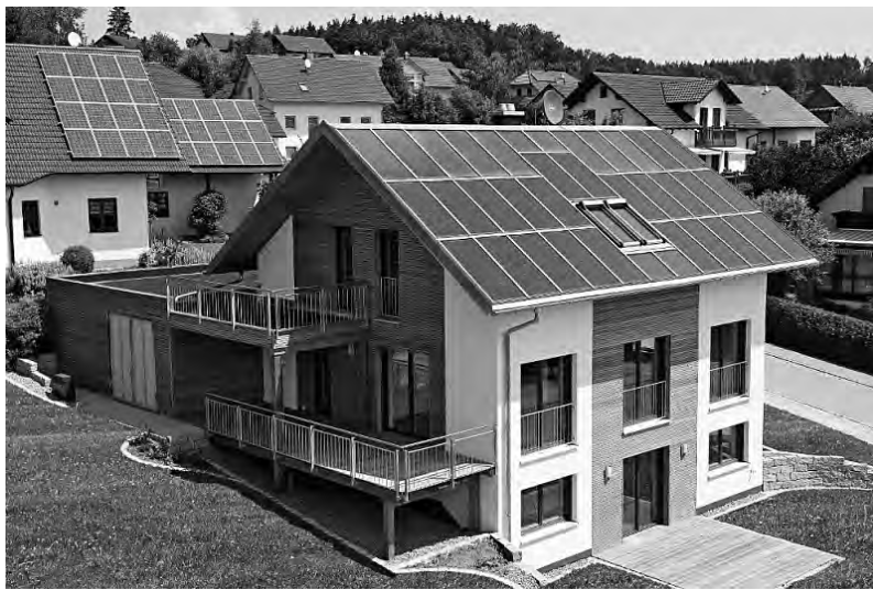
Fig. 1. Solar panels form the plane of the roof [9]
