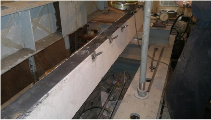
Fig. 4. Placing additional sheet reinforcement in the tension zone of the beam
