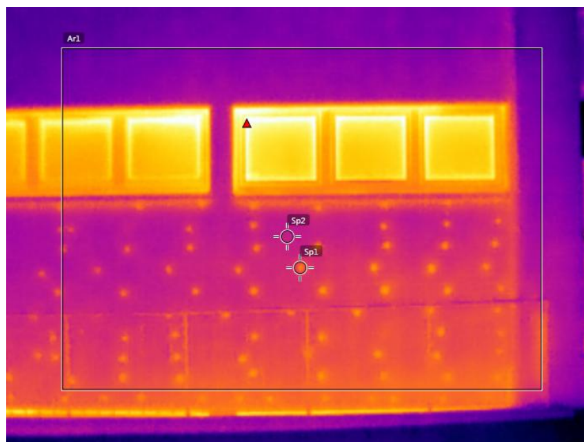
Fig. 1. Facade of the building after renovation, made by thermal imaging camera
