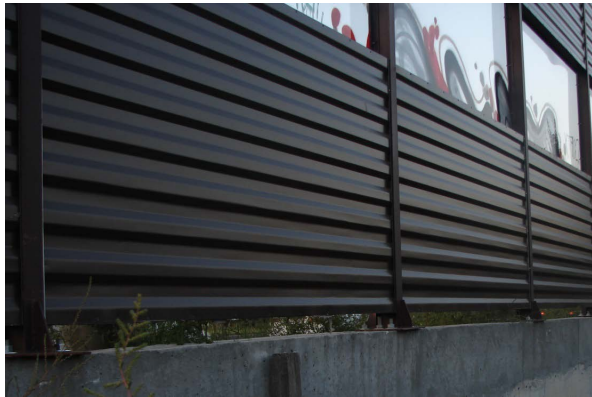
Fig. 1. A noise protection screen in the city of Kyiv, with a slit at its base
