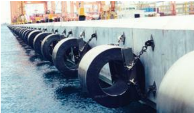
Figure 4 An example of an elastic hollow rubber bumper
