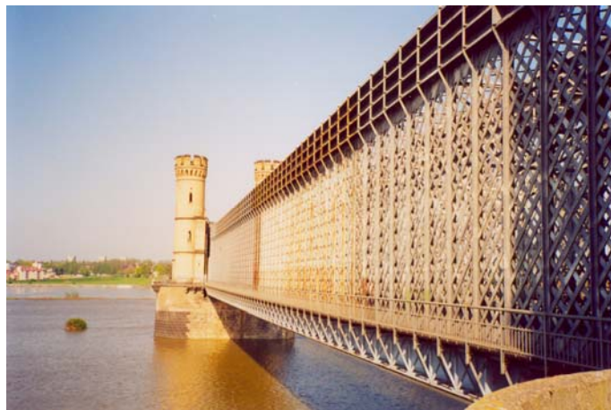
Fig. 5. The preserved Tczew Bridge original superstructure side view
