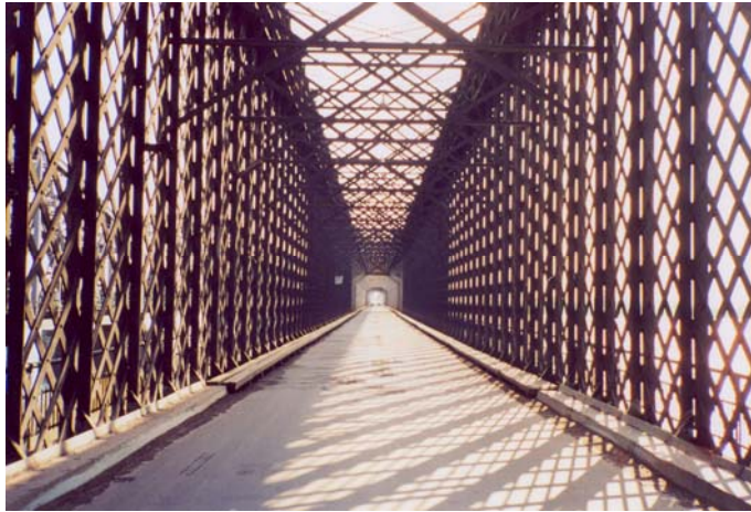
Fig. 6. The preserved Tczew Bridge original superstructure internal view
