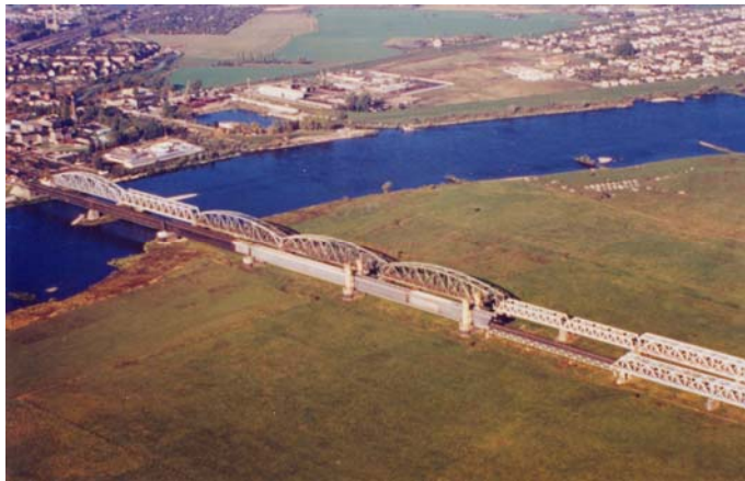
Fig. 7. Present aerial view of the Tczew bridges
