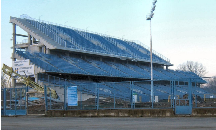
Fig.1. General view of tested structure of tribune
