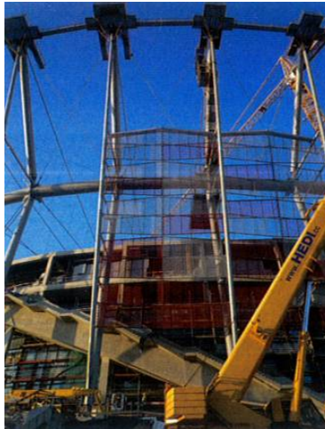
Fig. 19. Erection of the facade elements
