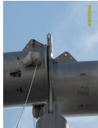
Fig. 10. The gap by closing ring
