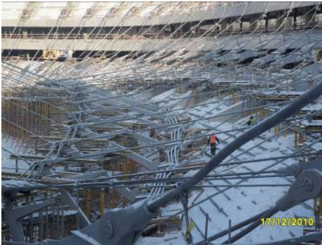
Fig. 12. Preparation of the cable roof to Big Lift
