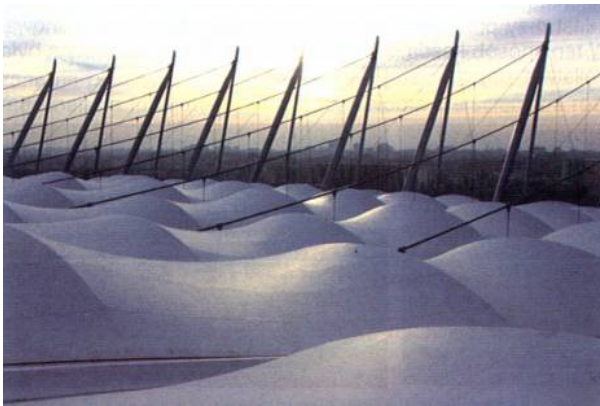
Fig. 15. The main roof – glass fibre cated by PTFE
