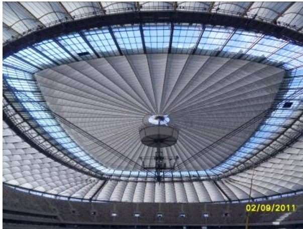
Fig. 16. Inner roof closed
