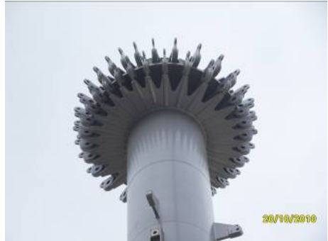
Fig. 6. Central knot seen downwards
