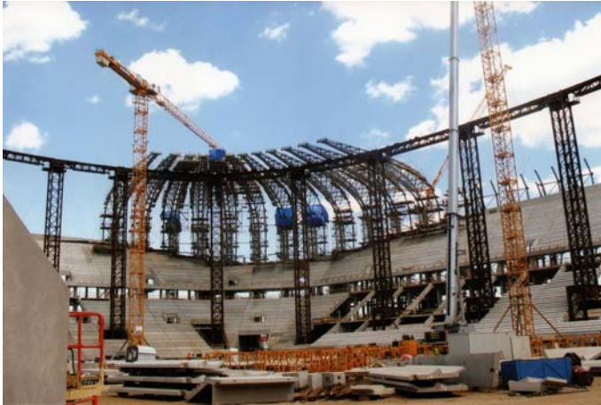
Fig. 20. Assembled 12 “roof” segments of the stand roofing carrying structure
