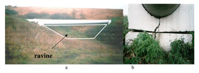
Picture 1 – Oil pipeline above ground crossing of the ravine: a – general view; b – destruction of concrete support
