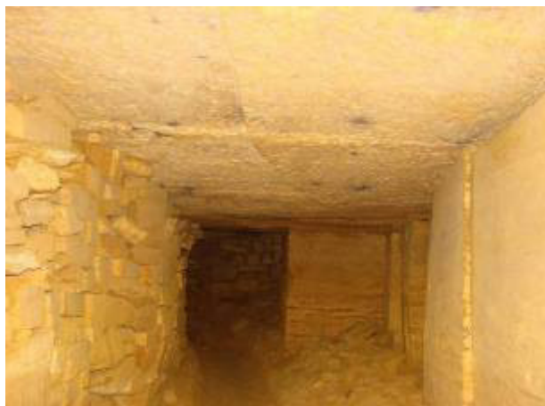
Figure 3 – General view of underground workings
