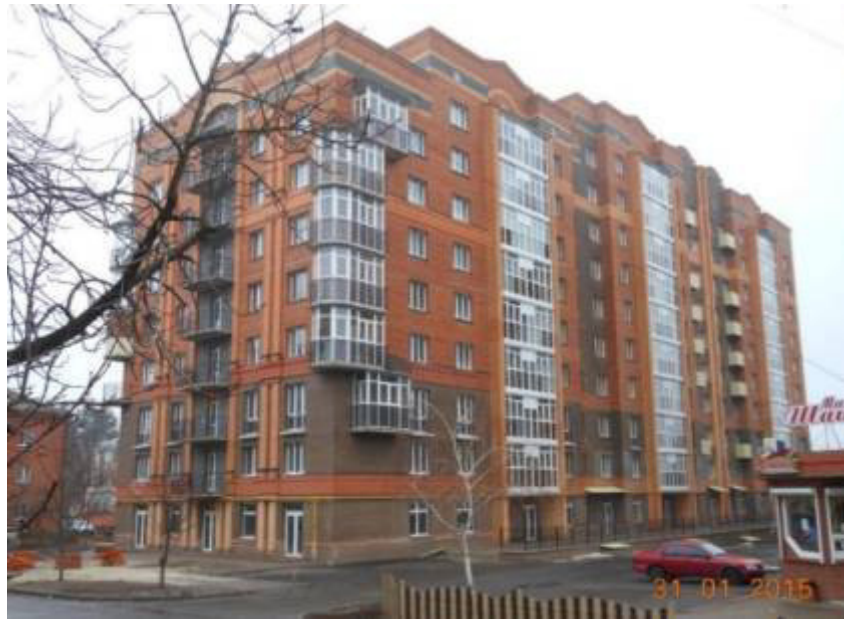
Figure 1 – General view of the three-sectioned nine-ten storey house in the str. V. Kozak, 14 in Poltava (order of sections – left – right)
