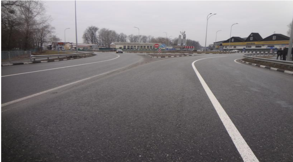
Figure 3 – General look, approach to the roundabout, Borodyanka
