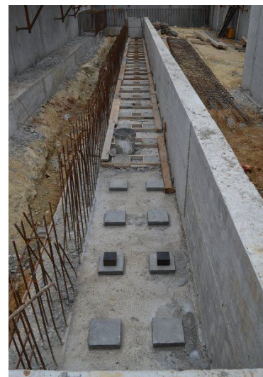
Fig. 4. Current construction status of the shock-tube slab.
