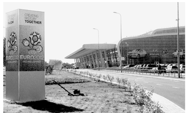
Fig. 21. New airport terminal. (© Bohdan Posatskyy, 2012)
