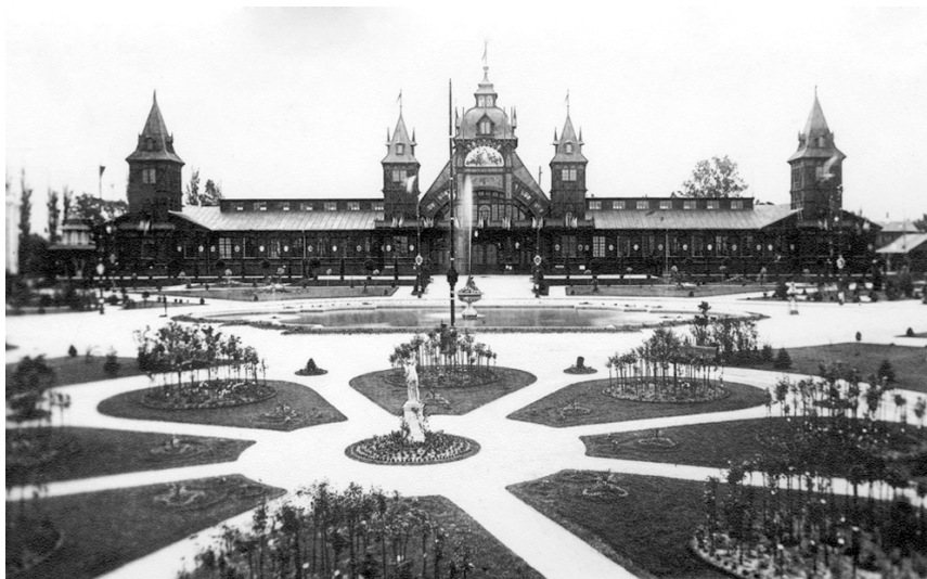
Fig. 5. Flower garden in front of the pavilion of industry at the Galician National Exhibition. Lviv, late 19 th century. Project by A. Röhring
