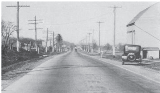
The first concrete Highway in New Jersey Built 1912, between Broadway and New Village
