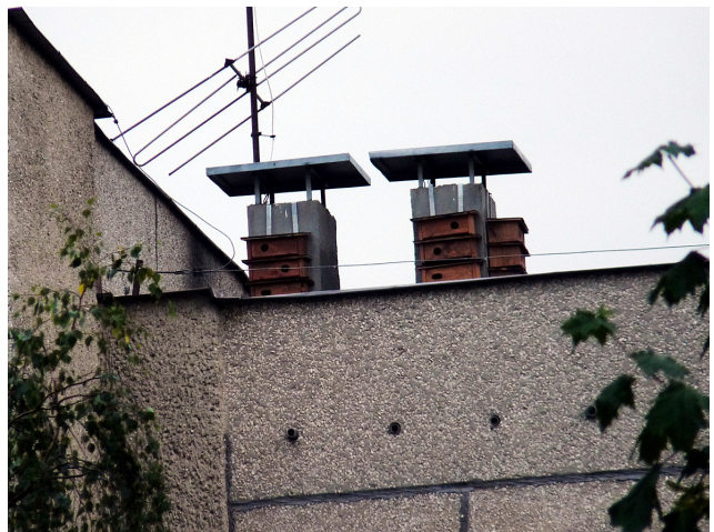
Fig. 10. Nesting boxes for swifts hung too low above the roof. There is no chance on their inhabiting by swifts
