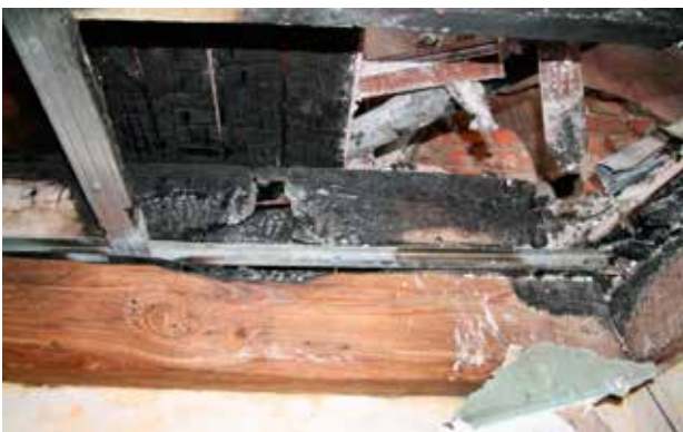
Ryc. 25, 26. Widok śladów ognia w źródle (fot. Tomasz Wiśniewski) Fig. 25, 26. Picture showing traces of fire in the ignition source (photos by Tomasz Wiśniewski)
