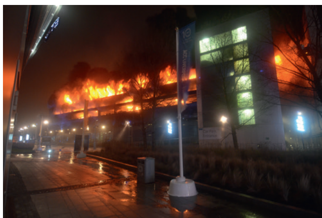
Figure 1. Fire at a multi-storey car park in Liverpool Source: Merseyside Fire & Rescue Service resources.
