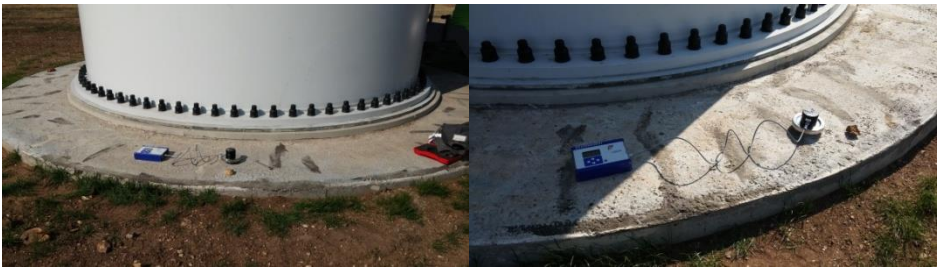
Fig. 5. Fixing a vibration indicator on WPU foundation
