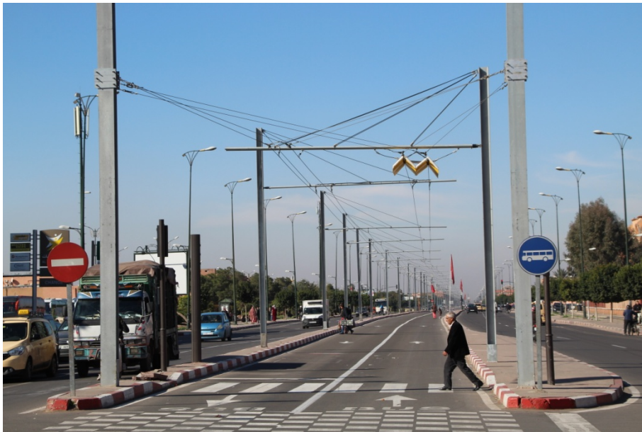
Fig.7. The eastern end of the catenary section of Marrakech's BRT system
