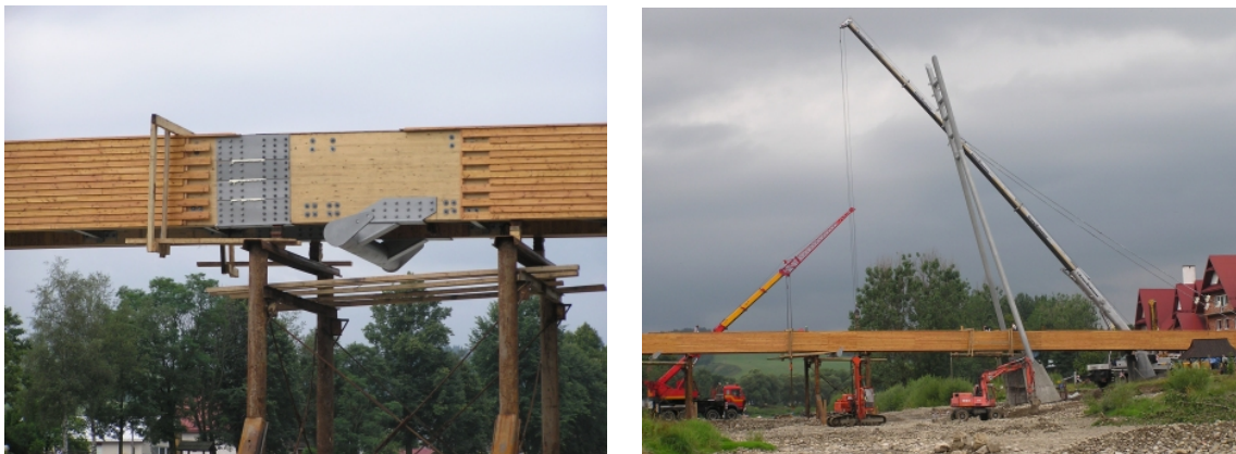
Fig. 7. Assembling of the footbridge deck on temporary supports (July 2006)
