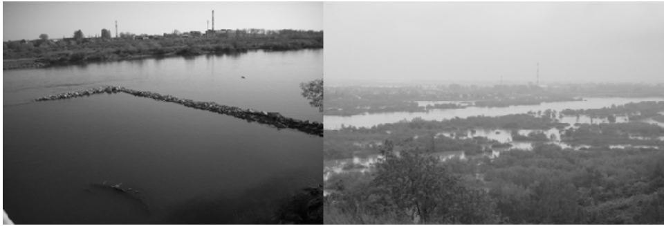
Phot. 1 – A Transversal Dam on the Vistula in Sandomierz and the Inter-Embankment Zone within the Town’s Territory Covered with Wicker, Bushes and Trees
