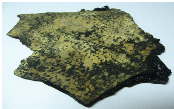
Figure 7 – Photo of the damaged bituminous coating
