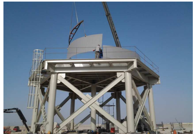
Figure 2 – General view of storage constructing process made in Saudi Arabia
