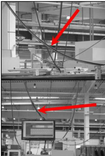
Figure 7. Not professional assembly of el. cable
